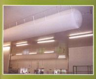
Trevira says its polyester fibre, CS Bioactive, has several advantageous properties when used to make the fabric for these heating, ventilation and air-conditioning ducts 8
